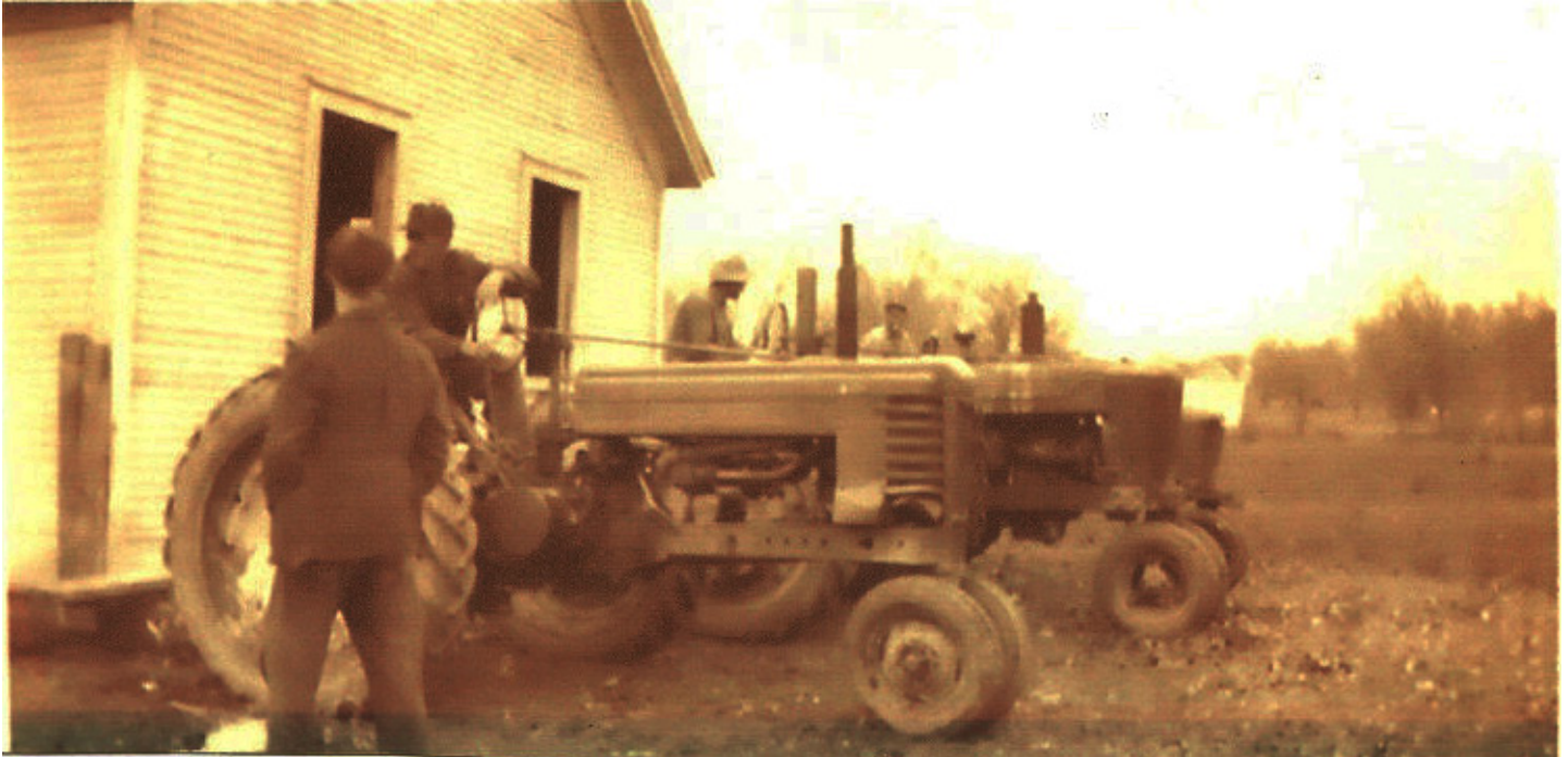
Above: Moving the old schoolhouse to its present location where it serves as the town hall.
