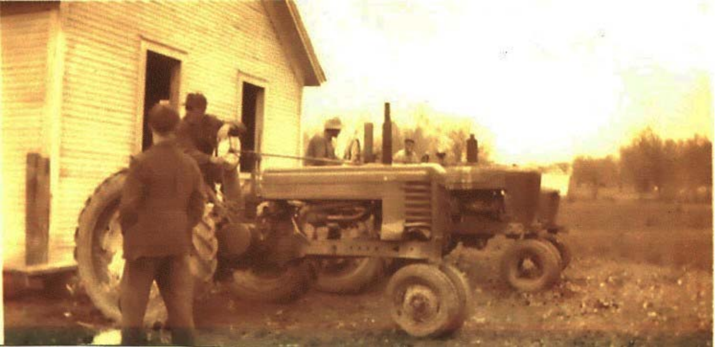
Above: Moving the old schoolhouse to its present location where it serves as the town hall.
